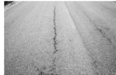
First stage of wheel path cracking caused by heavy traffic loads.
